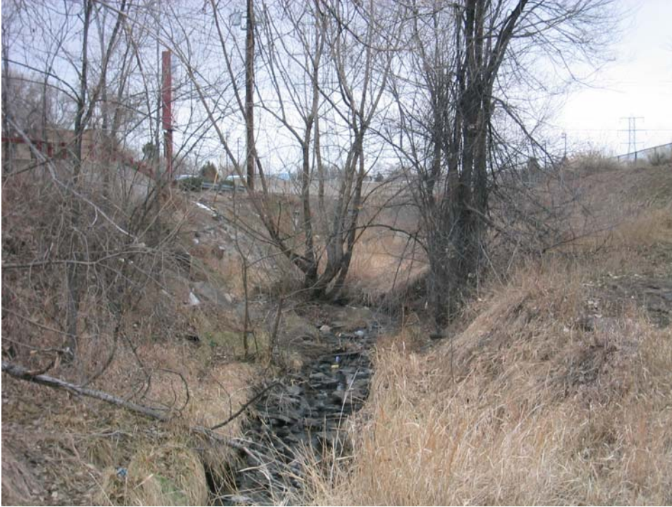
2. Dry Gulch drains through property
