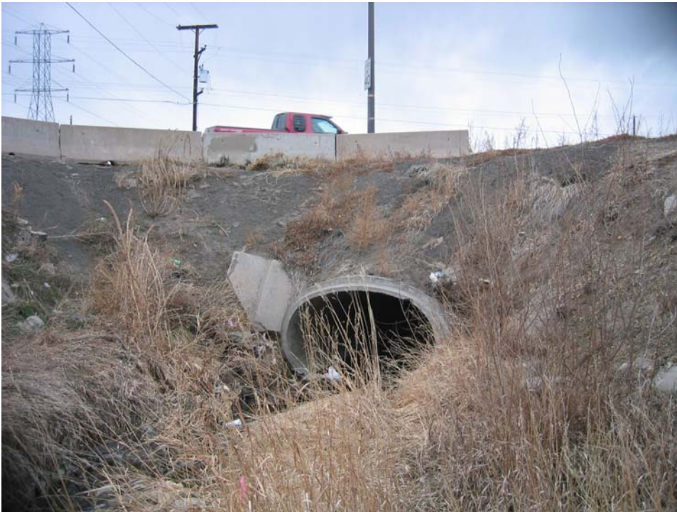
3. Existing culvert outfall at western boundary of property
